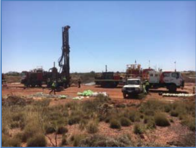
Bibra RC Drilling Operations
