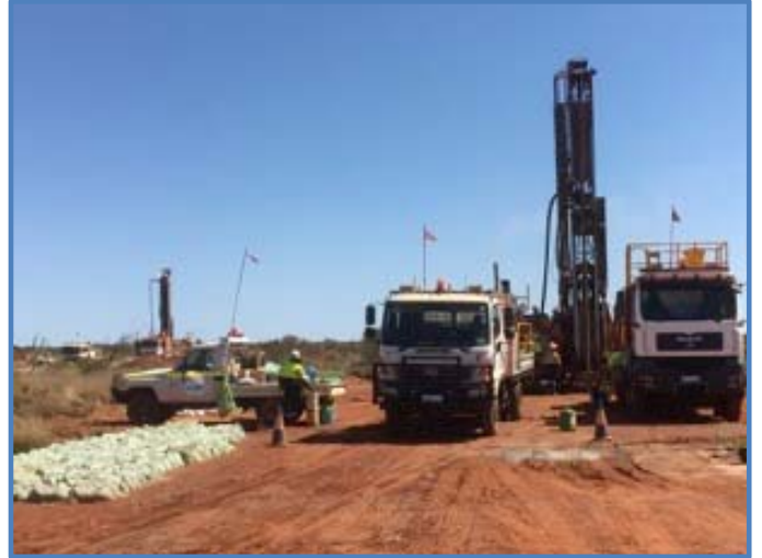
Bibra RC Drilling Operations
