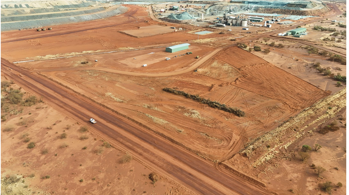
Karlawinda Expansion Project – Early Clearing Works
