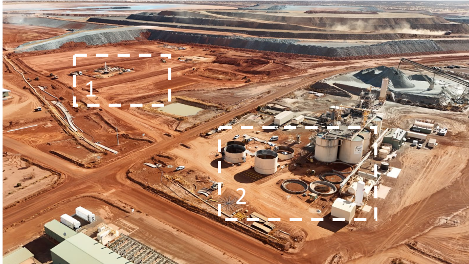
KEP Processing Plant Site
