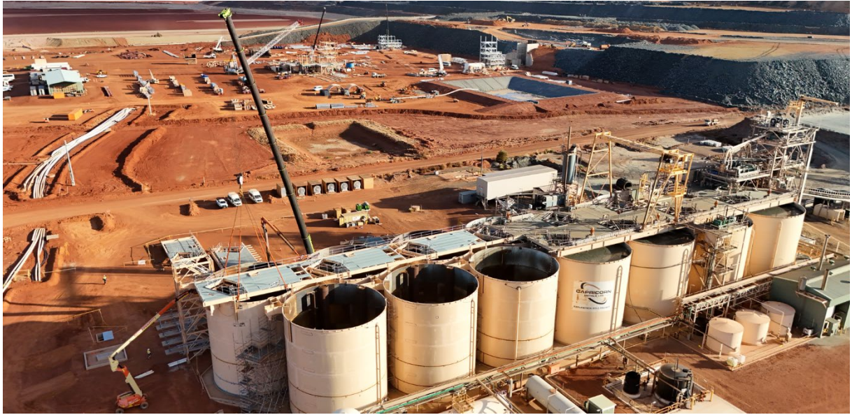
Karlawinda Expansion Project – CIL circuit extension with top of tank steel sections being lifted into place.
